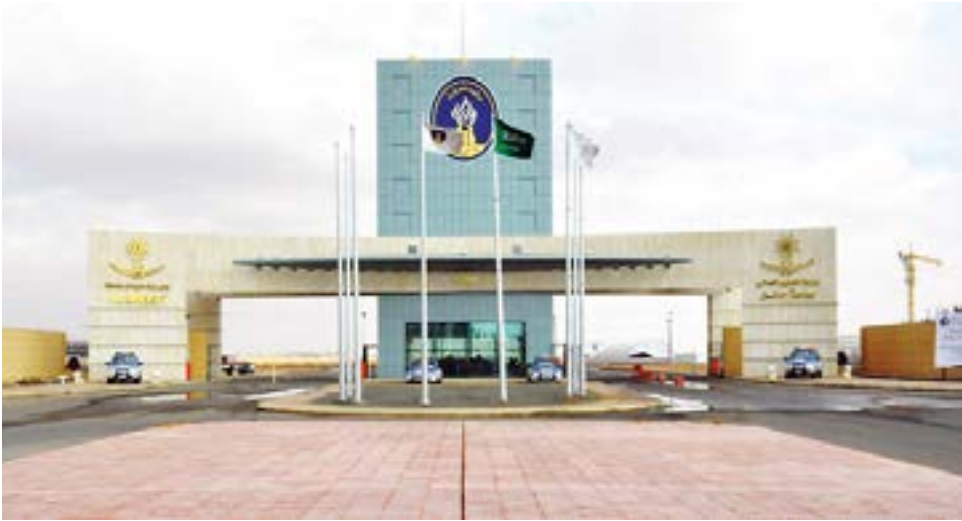
Project: Hail University Site Development & Infrastructure Hail, KSA
