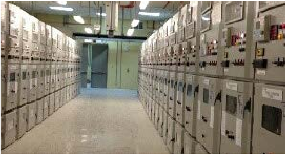
Project: Construction of 110/13.8kV Arafat-2 Substation Makkah, KSA
