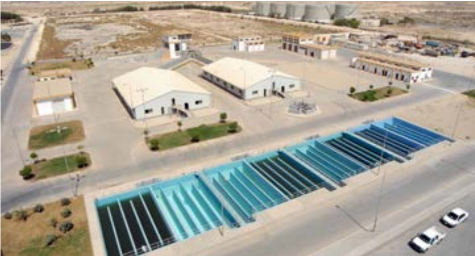
Project: Sewage Treatment Plant Quatif, KSA
