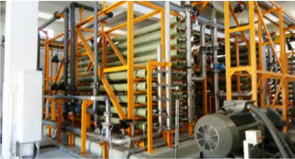
Project: Wadi Aldwaser Water Treatment Plant
