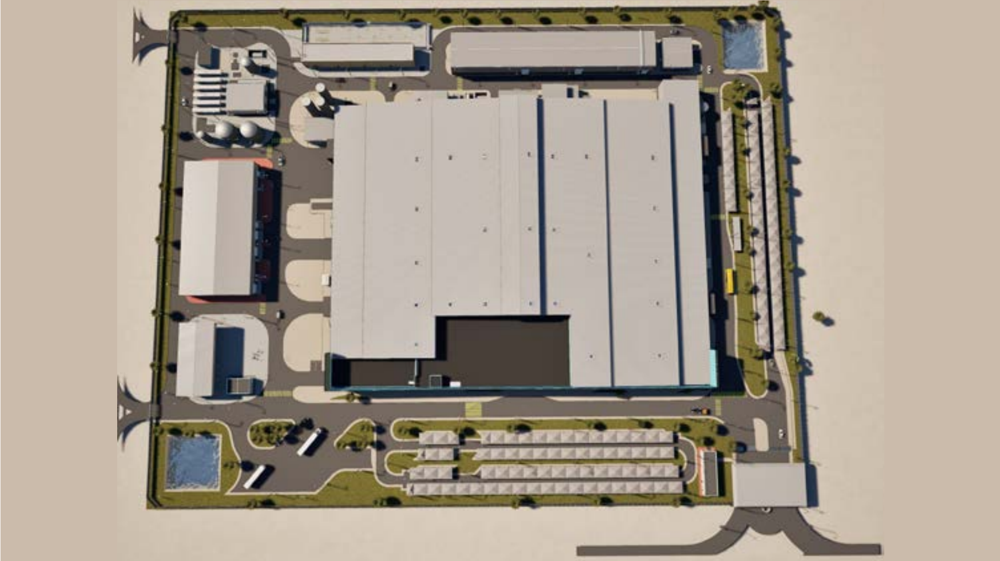
Project: Mechanical Services Shops Department (MSSD)– Aerial View
