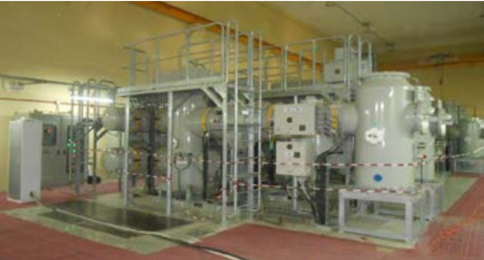
Project: Construction of 110/13.8kV Al-Zahra-2 Substation Makkah, KSA
