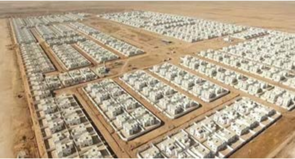
Project: Infrastructure Development of Northern Housing Tabouk, KSA
