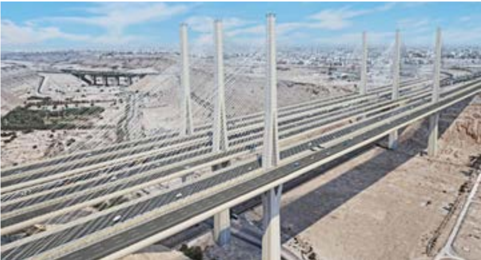
Project: Wadi Laban Bridge Riyadh, KSA
