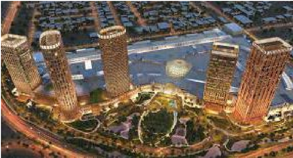
Project: The Avenues – (Towers 1 & 3) Riyadh, KSA
