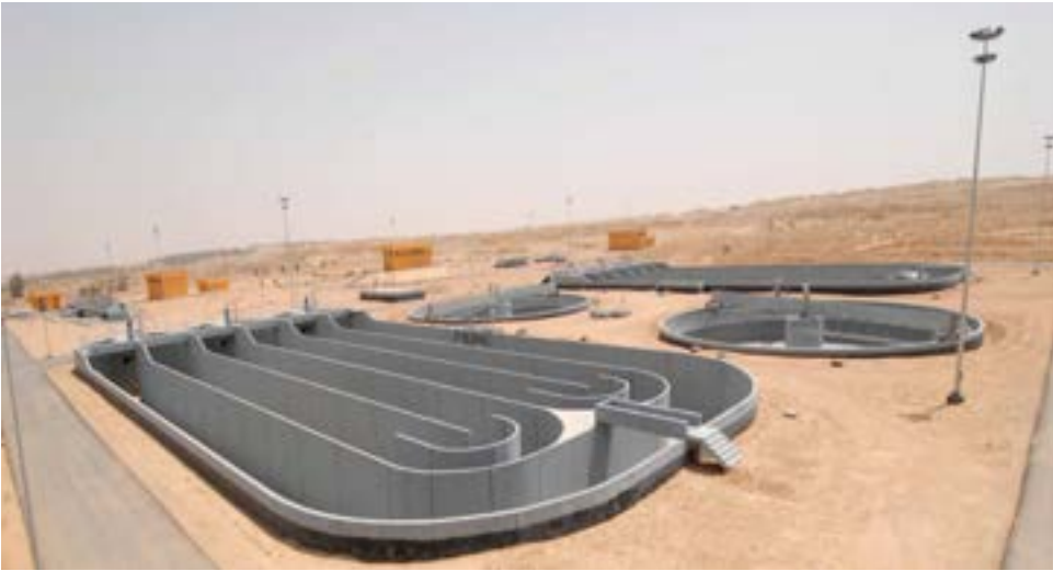
Project: Sewage Treatment Plant Unyazah, KSA
