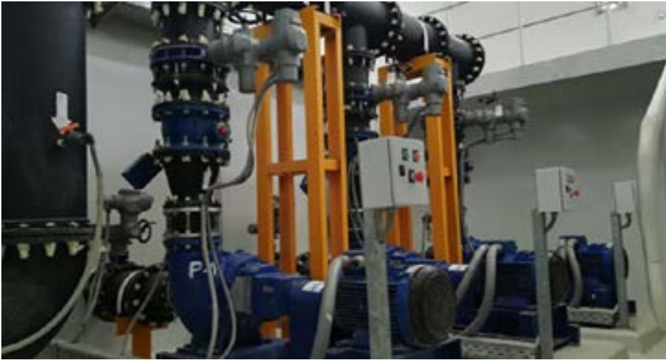
Project: Najran Water Treatment Plant Najran, KSA
