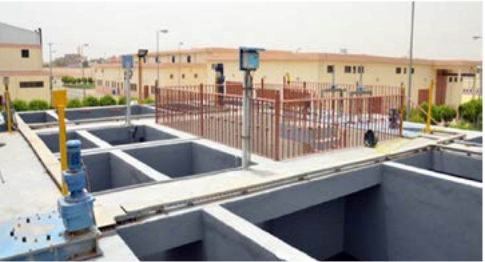
Project: Beyesh Water Treatment Plant
