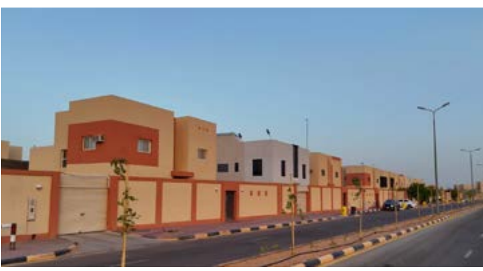
Project: Infrastructure Development of Northern Housing Sakaka, KSA
