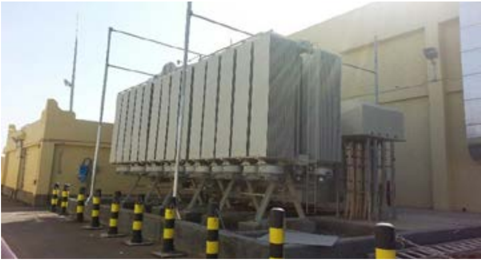
Project: Construction of 110/13.8kV Wali Al Ahad Substation Ras Al-Khair, KSA
