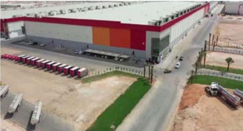
Project: Agility Logistics Hub (40,000 m³) Riyadh, KSA
