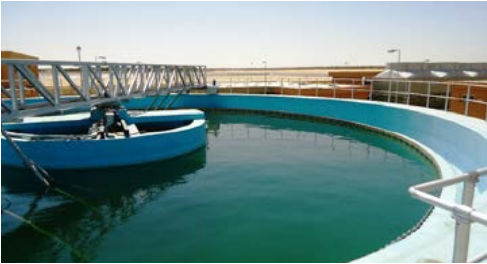
Project: Najran Water Treatment Plant Najran, KSA
