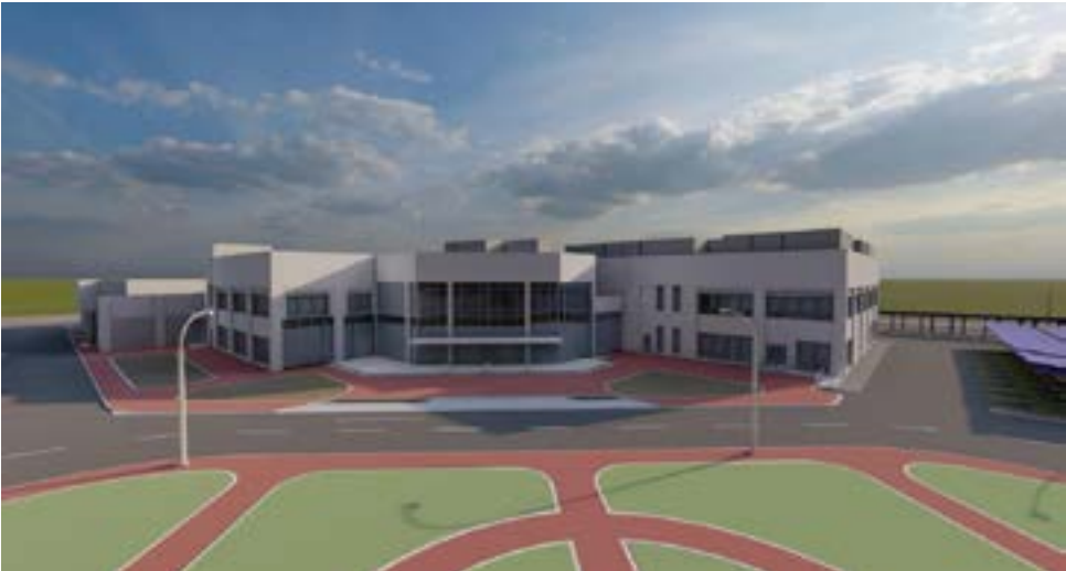
Project: Aramco Package 6 – Amiral Industrial Support Facilities – Petrochemical Lab Building
