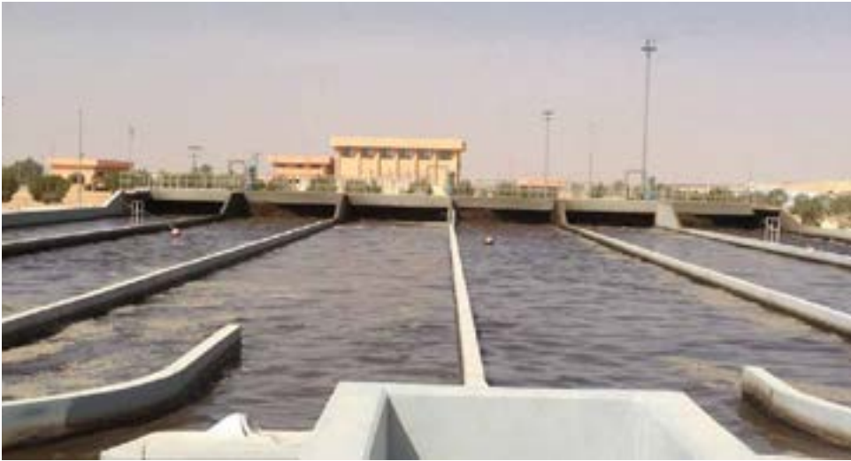
Project: Sewage Treatment Plant Unyazah, KSA
