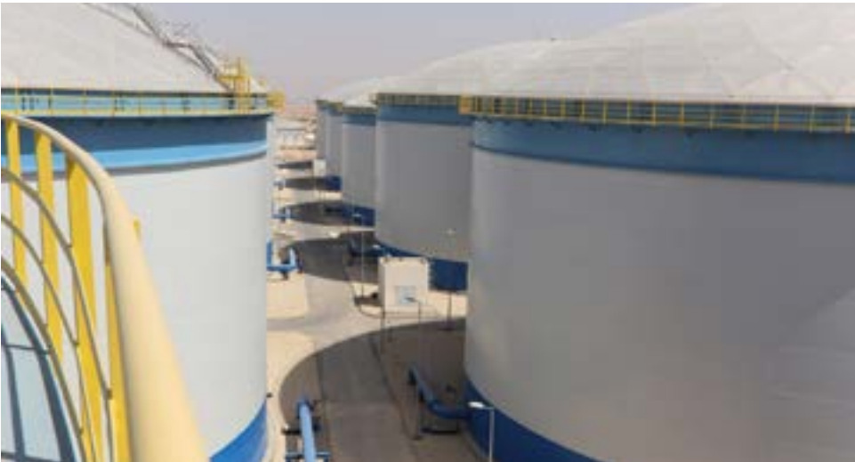
Project: Riyadh Strategic Water Reservoirs (20,000 m³) Riyadh, KSA
