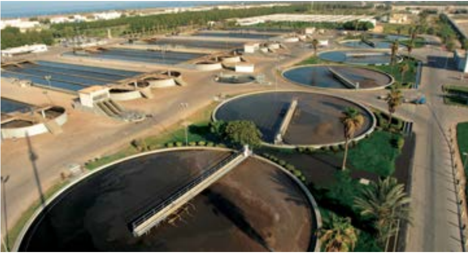
Project: Waste Water Treatment Plant Al-Khobar, KSA
