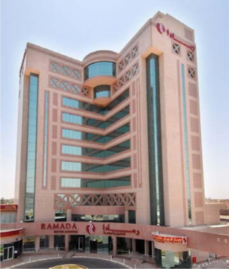
Project: Ramada Hotel AlQassim, KSA
