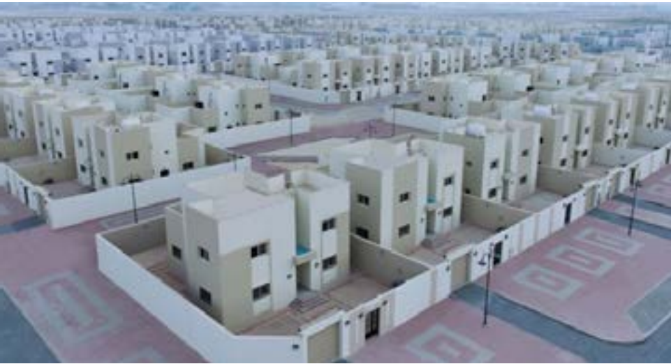
Project: Infrastructure Development of Eastern Housing AlKhobar, KSA
