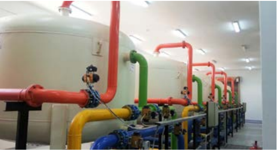
Project: Wadi Aldwaser Water Treatment Plant
