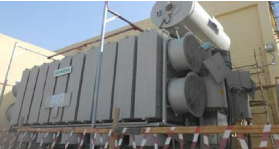
Project: Construction of 110/13.8kV Al-Zahra-2 Substation Makkah, KSA
