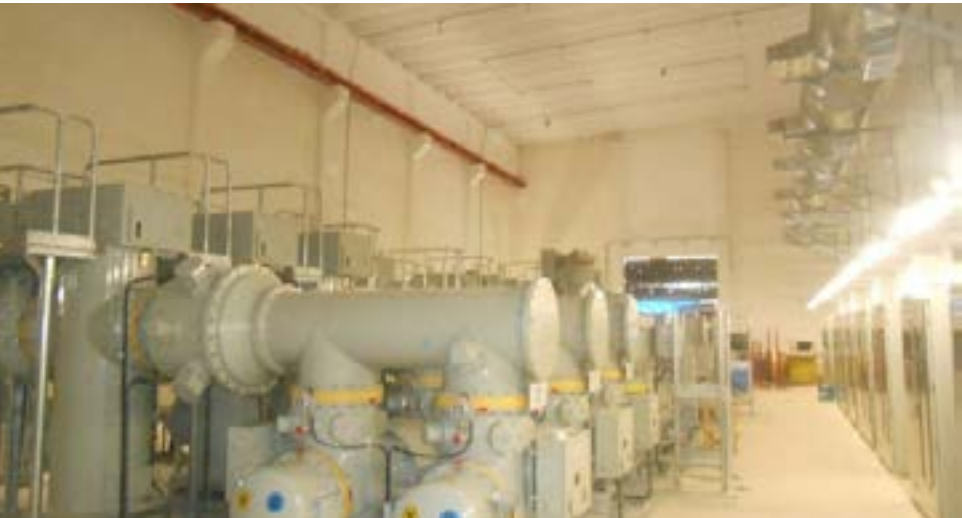
Project: Construction of Nimar 132/13.8kV Substation # 8132 Riyadh, KSA
