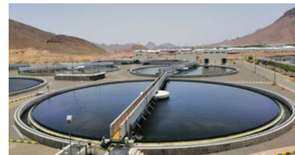
Project: Main sewage treatment plant 2_nd phase
