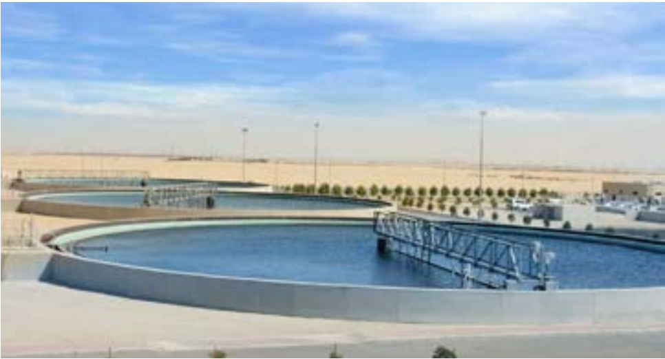
Project: Beyesh Water Treatment Plant
