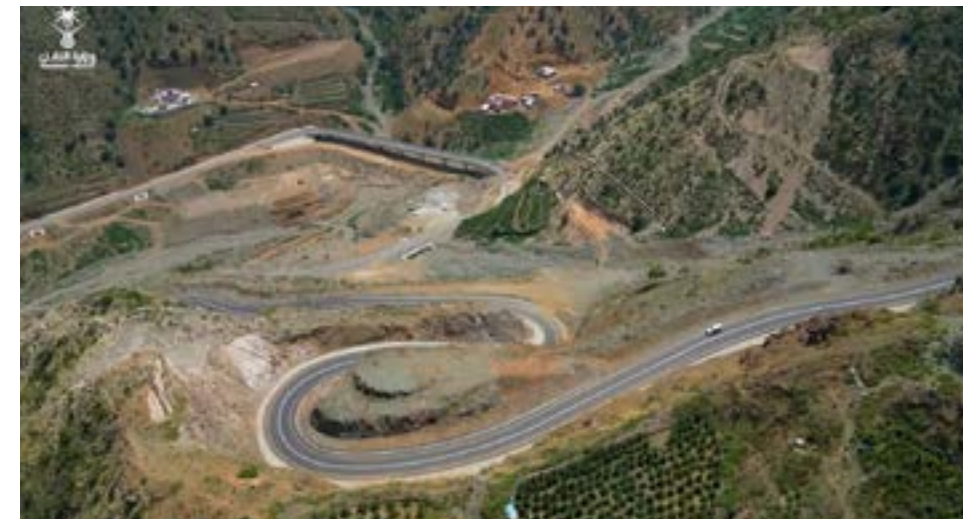
Project: Upgrading of Road ways Group 14
