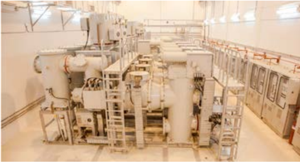
Project: Construction of New 110/33/13.8 kV Badr Substation Badr Area, KSA
