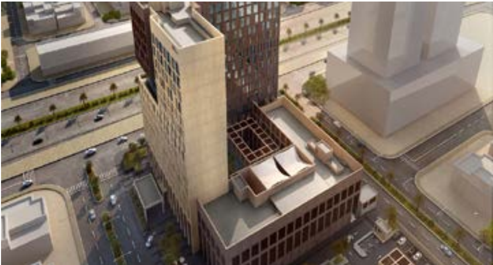
Project: Mawten Tower – Hilton Complex (50,000 m³) Riyadh, KSA
