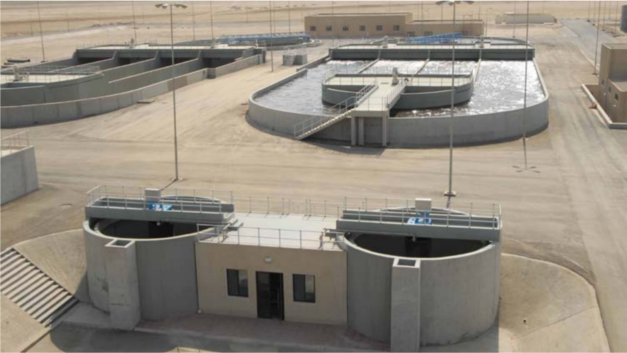
Project: Sewage Treatment Plant
