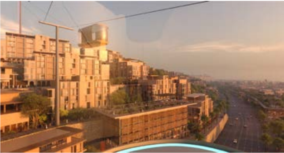
Project: Corniche El Mokattam - Guest Village
