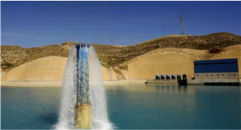
Project: Damad Sewer Networks
