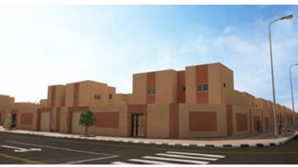
Project: Infrastructure Development of Northern Housing Turaif, KSA
