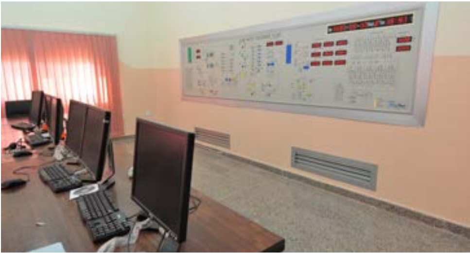
Project: Damad Sewer Networks
