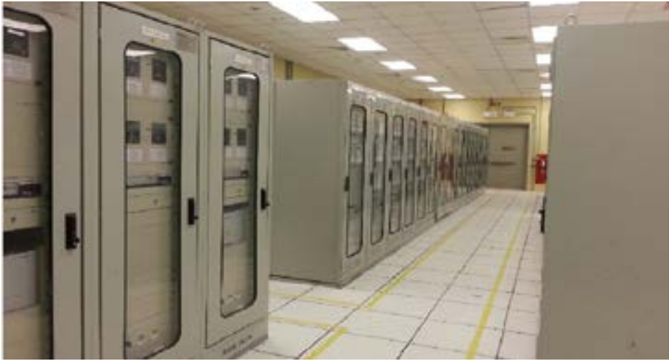
Project: Construction of Almansourah 132/13.8kV Substation # 8186 Riyadh, KSA
