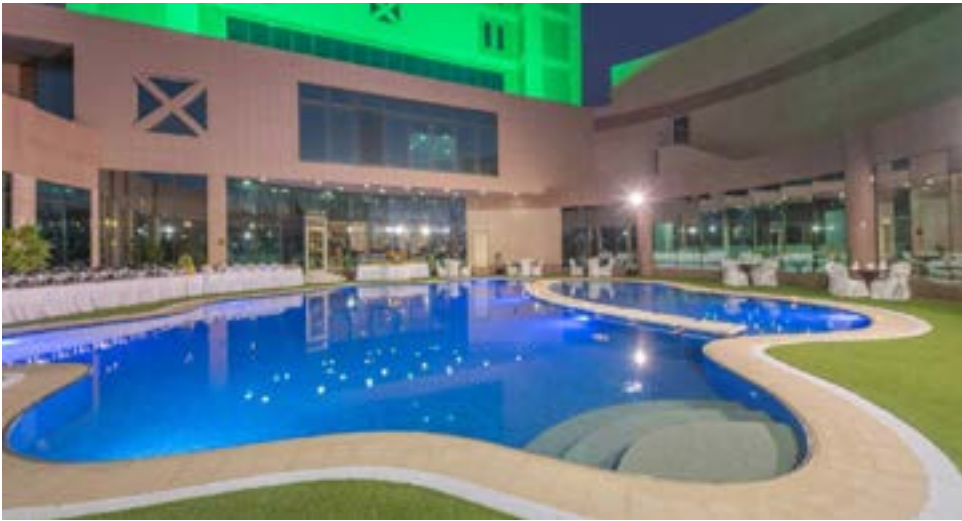
Project: Ramada Hotel AlQassim, KSA
