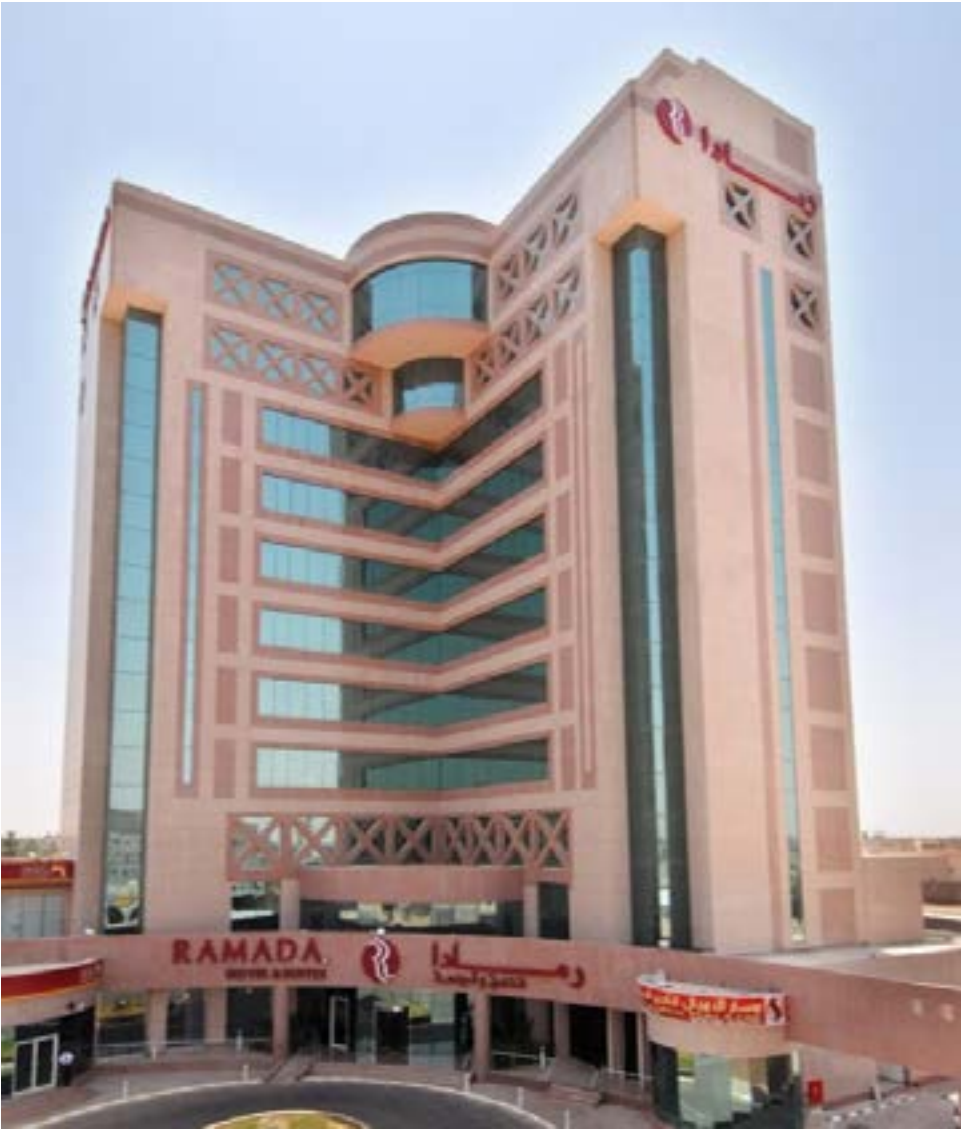
Project: Ramada Hotel AlQassim, KSA
