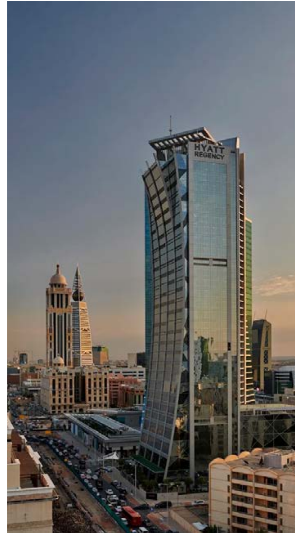
Project: Al Swailem Tower Hayatt Regency Hotel
