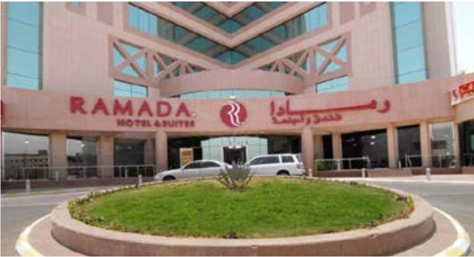
Project: Ramada Hotel AlQassim, KSA
