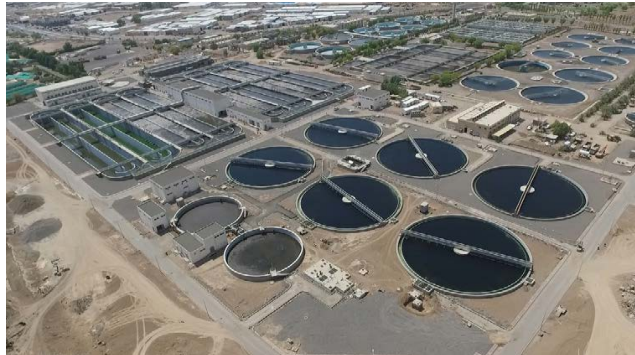
Project: Main sewage treatment plant 2_nd phase
